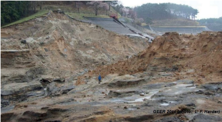
↑ Figura 7. Restos de la presa Fujinuma después del sismo de Tohoku (tomada de Preliminary Observations of the Fujinuma Dam Failure Following the March 11, 2011 Tohoku Offshore Earthquake, Japan (p. 9), por Leslie F. Harder, 2011, Geotechnical Extreme Events Reconnaissance).
