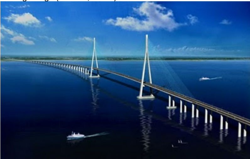
Sutong Bridge (Suzhou, China)
