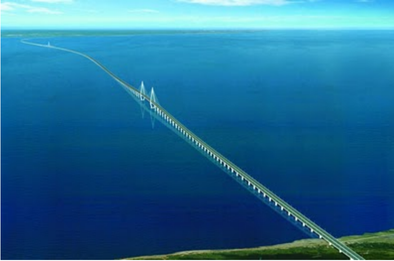
Donghai Bridge (Shanghai, China)
