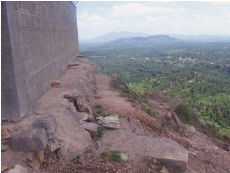
Figure 9.5 Discordant constructions at the peak (Murithi 2011)
