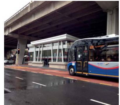
MYCITI BUS AND FEEDER STATION, GARDENS
