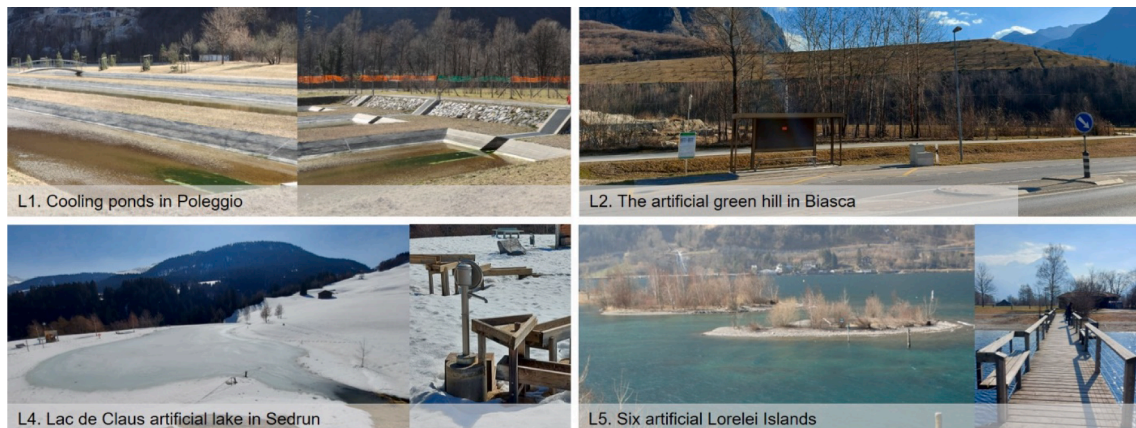
Fig. 10. Some ecological and hydraulic compensation works at the local level of the Gotthard System (Source: Authors).
