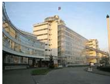
Van Nelle Factory, designed by Johannes Brinkman and Leendert van der Vlugt, 1931, Rotterdam. Photo: Kyle Normandin
